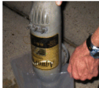
Step 6 - Remove from bag, flush contents to sewer, dispose of bag and re-install
