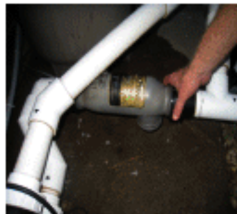
Step 1 - Remove Salt Cell Chlorinator from System
