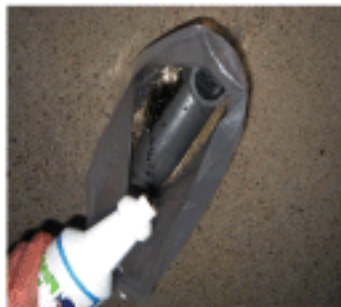
Step 4 - Add 1 - 32 oz. bottle of Piranha Salt Cell Cleaner to water
