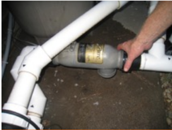
Step 1 – Remove Salt Cell Chlorinator
